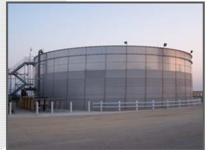
Bolted Stainless Steel Tank
