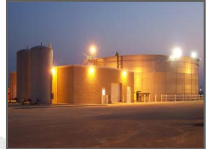
HRAS Treatment Plant
